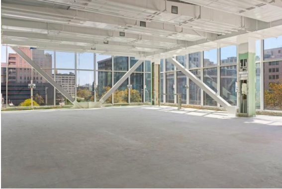
Studio in Colburn's new Frank Gehry-designed Dance Center under construction in Downtown.
